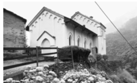
Waldenserkirche in Torre Pellice, Piemont. Foto: Adobe Stock
